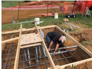
Figure 4b. Rebar Reinforced
